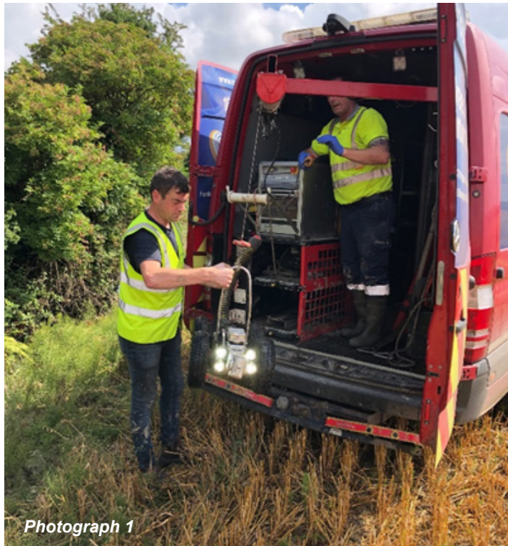
Photograph 1 is showing the survey contractor getting the equipment ready for the survey. Photograph 2 is showing the survey contractor conducting the CCTV survey of the culverts.
